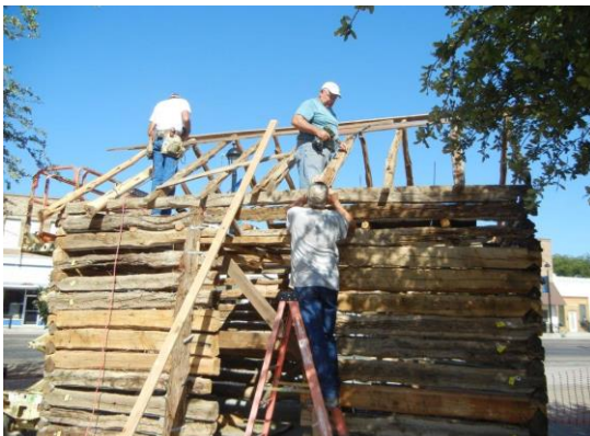
Starting the Roof
