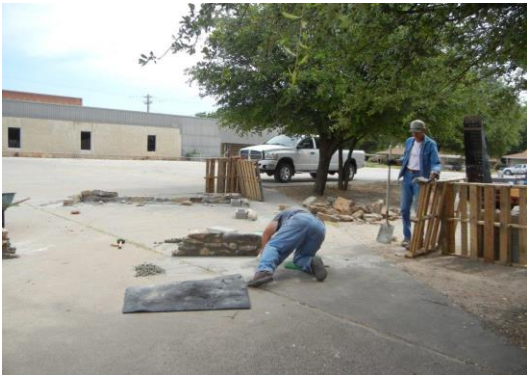
Laying New Foundation
